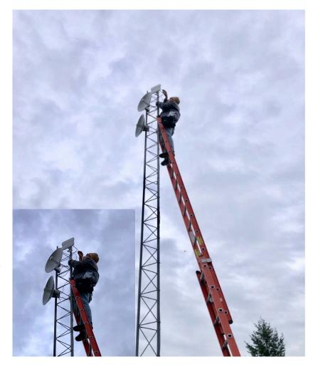
Nate was installing a new, slightly modified radio on the tower that allowed us to analyze the interference pattern real-time. Having this ability allowed us to then go to each affected client radio site and successfully adjust them to eliminate the interference. This actually also increased the bandwidth delivered to those three clients!
